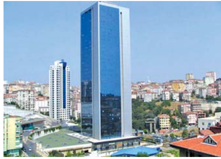
Polat Towers Residence, İstanbul
