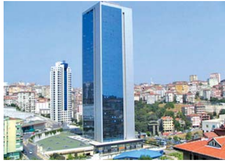
Polat Towers Residence, İstanbul
